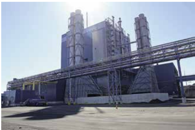
Outokumpu's new ferrochrome plant in Tornio Photo: Outokumpu
